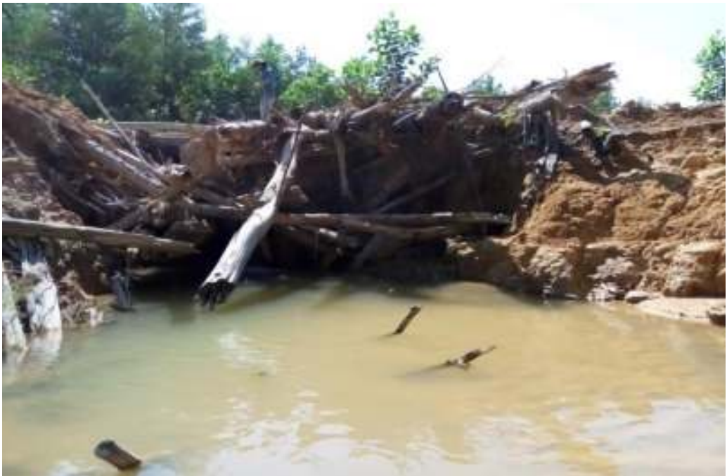
Figure 18. Logs piled as a crossing bridge blocks river flow
